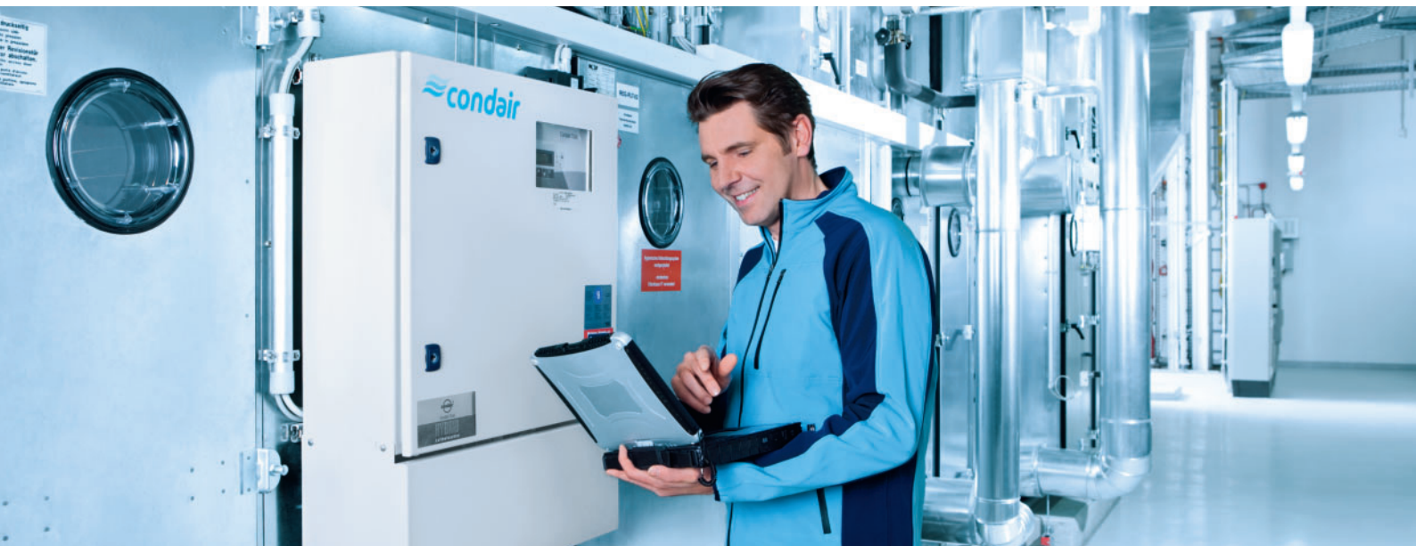
Condair Dual in an air handling unit (AHU)
